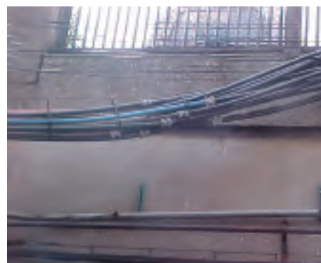
Transition from Aerial to LSZH using Split-Lock coupler.
